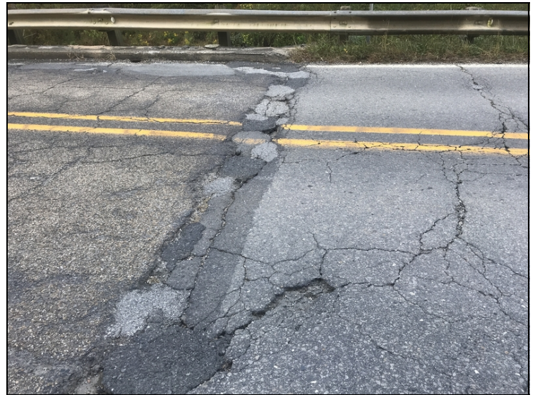
North asphalt approach has settled 2" and has potholes at abutment.
