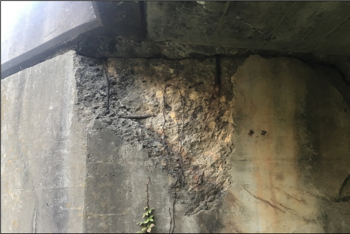
Bent 3 abutment has spall with exposed rebar on left side of girder 1.
