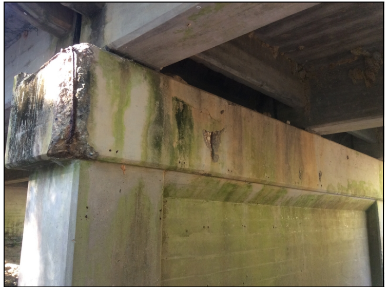
Bt. 2 ahead, right side, exposed rebar.
