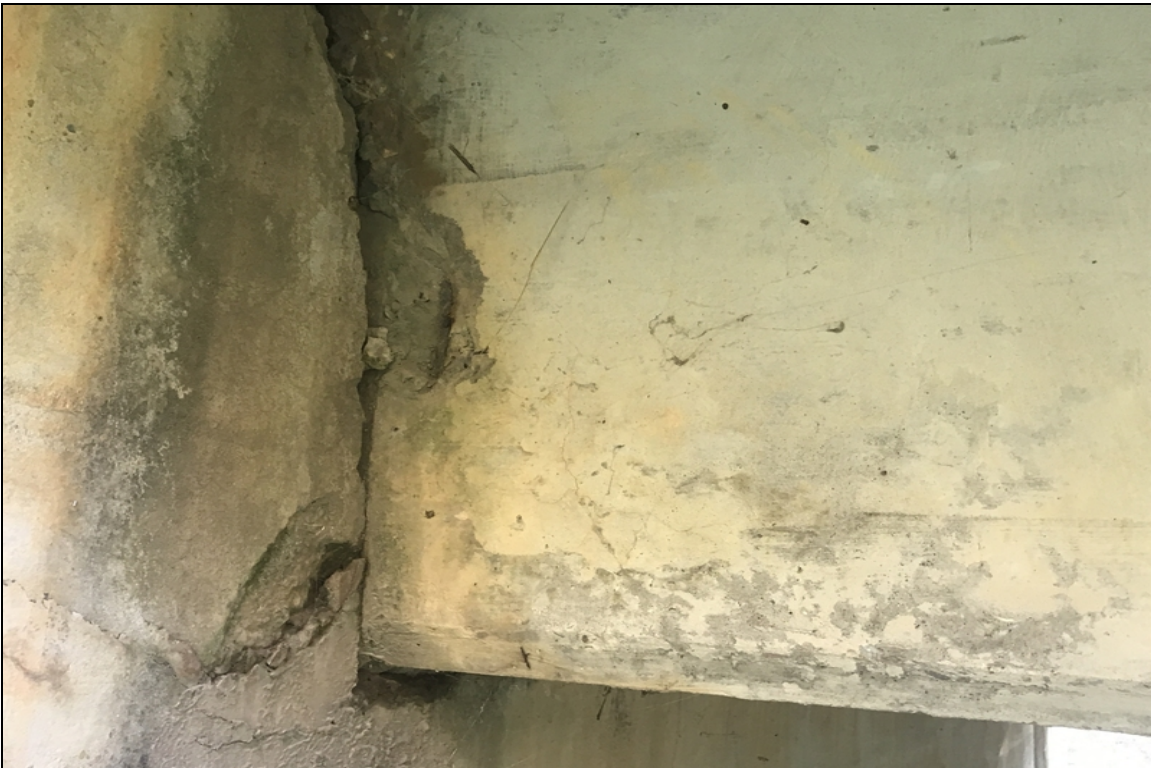
Girder 1 span 2 at bent 3 has spall with exposed rebar.
