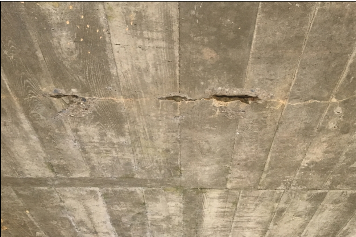
Span 1 soffit left of girder 2 has spall with exposed rebar.
