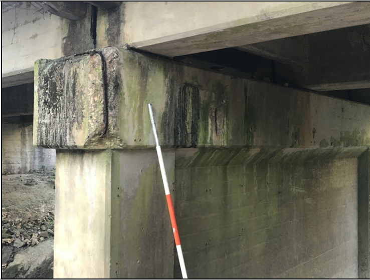
Bent 2 cap has spalls with exposed rebar.
