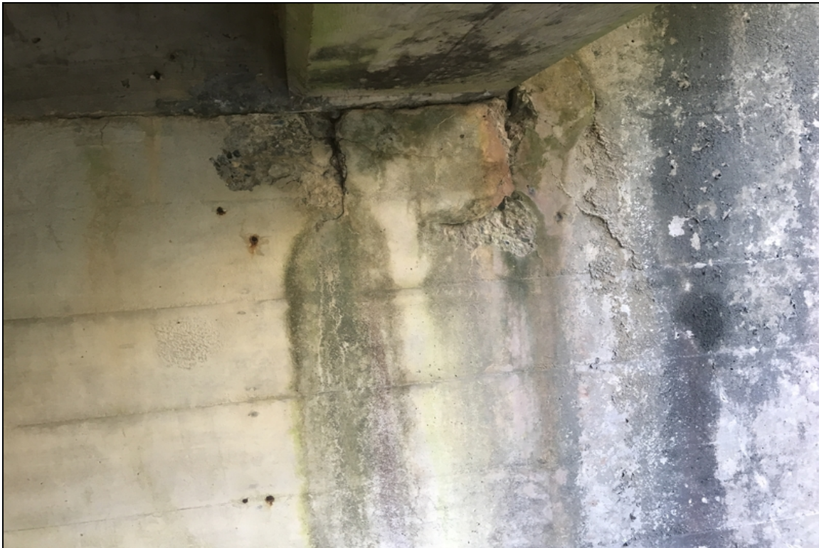
Bent 1 abutment has delam under beam 1.
