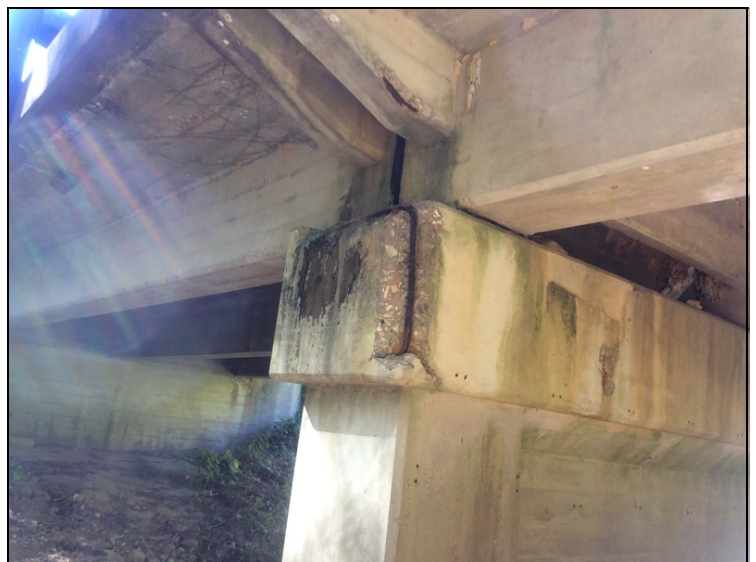
Exposed rebar
