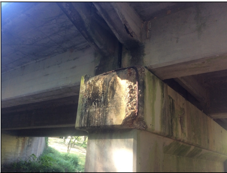
Bent 2 right side, spall with exposed rebar.
