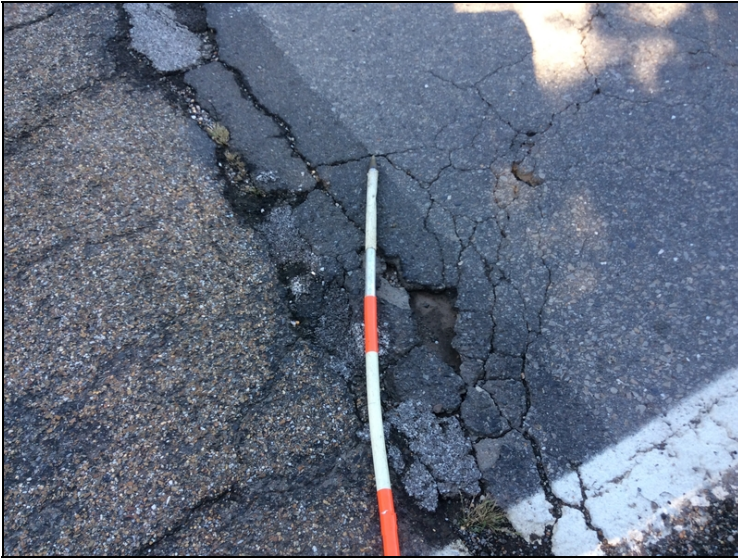
Potholes at the north end of the bridge.
