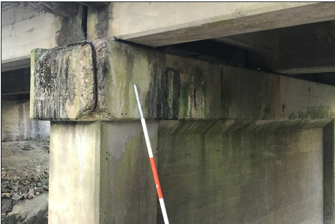
Bent 2 cap has spalls with exposed rebar.
