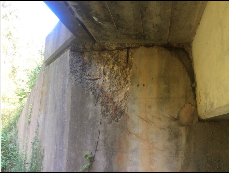
Bent 3 left side, large spall with exposed rebar.
